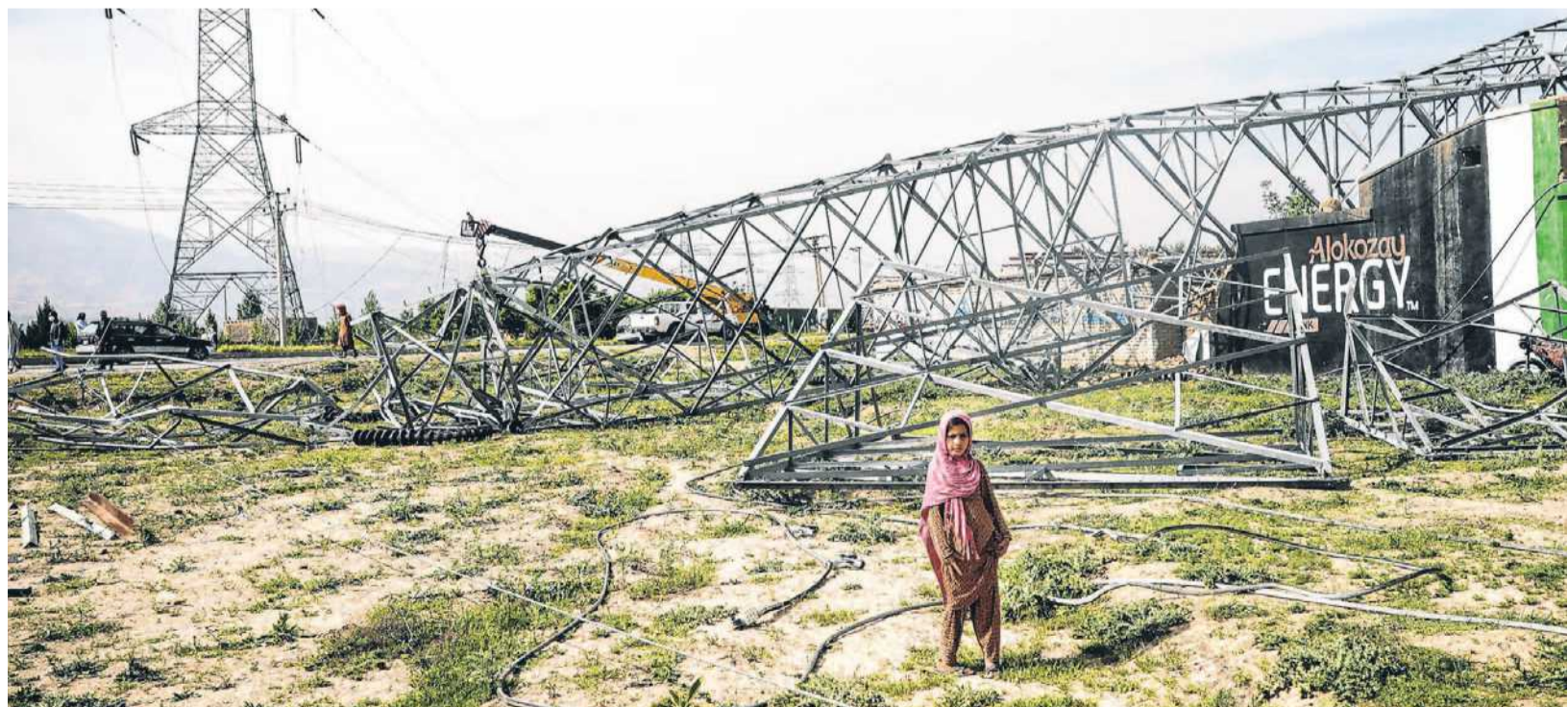
POWER WOES: A damaged pylon on the outskirts of Kabul, Afghanistan. The capital city has experienced severe power cuts after militants recently bombed equipment.
